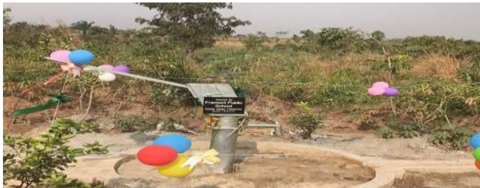
Commissioning of the newly drilled borehole by Rev. Fr. Peter Omogo for SOF.
